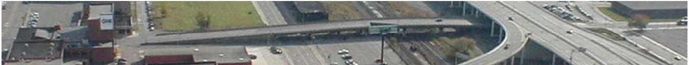
Michigan Street Bridge over Exchange Street and CSX Railway City of Buffalo
